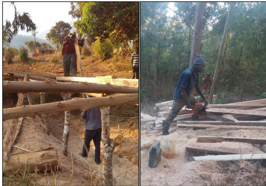
Figure 13.1 Pit and chain sawing
