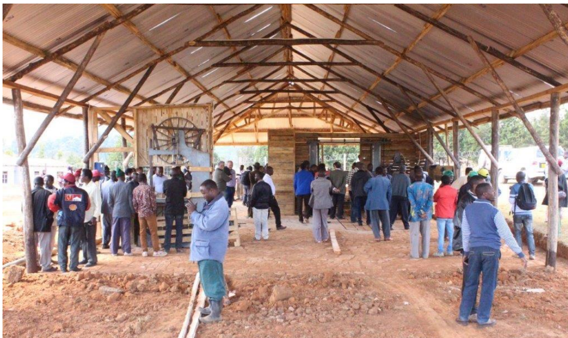
Figure 34 Opening of the newly established sawmill facilities in Makete industrial node
